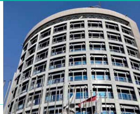
The Bank's HQ in Cairo, Egypt
